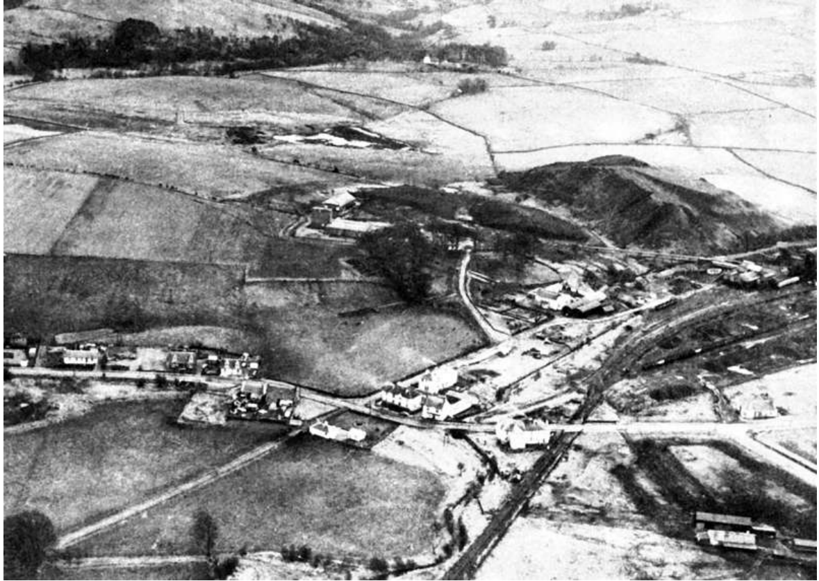
Aerial view of Connel Park shortly after the 'raws' were demolished
